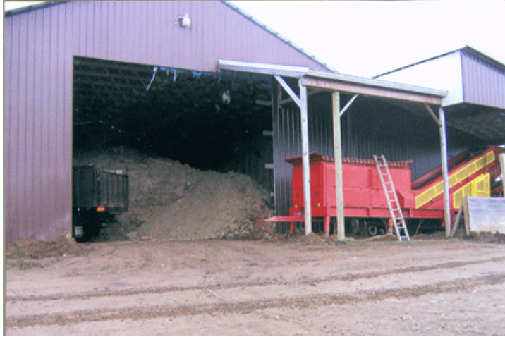
Existing dry building
