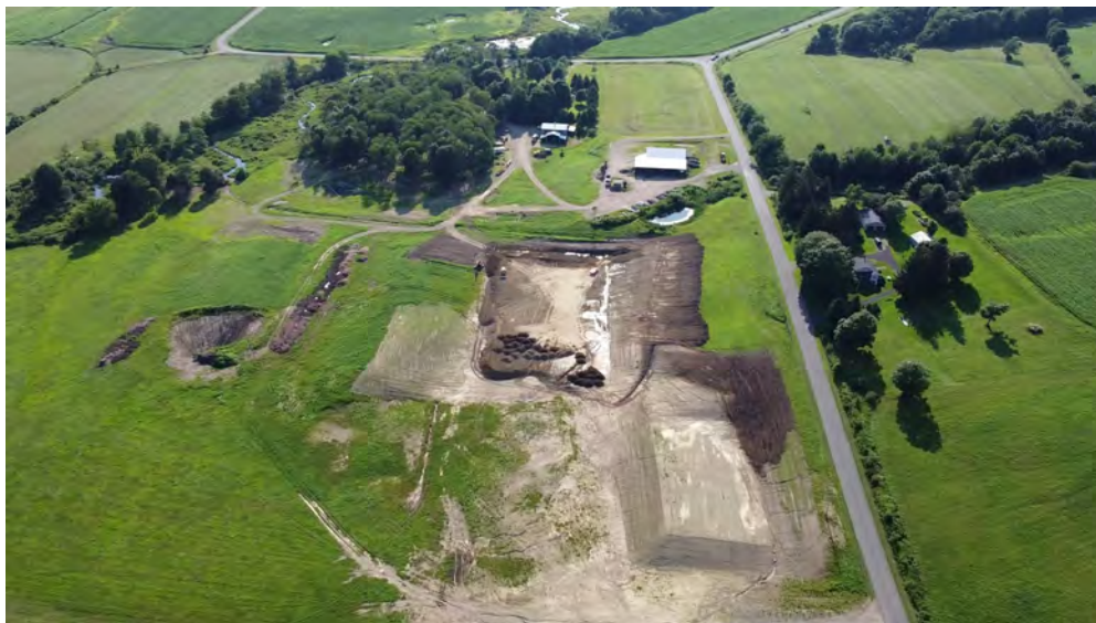
Images 20-23: Expansion site-work for future compost building
