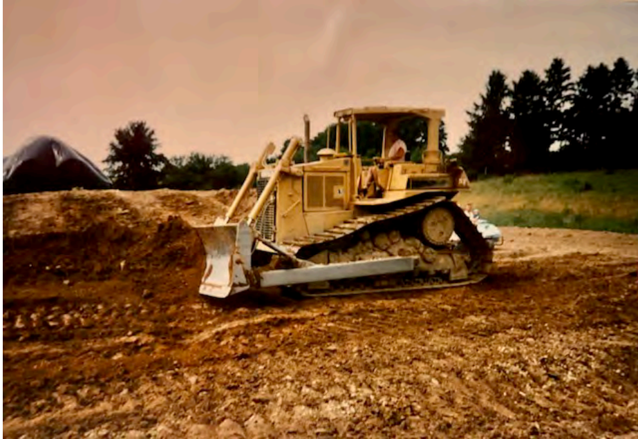
1992: Breaking ground for dry building
